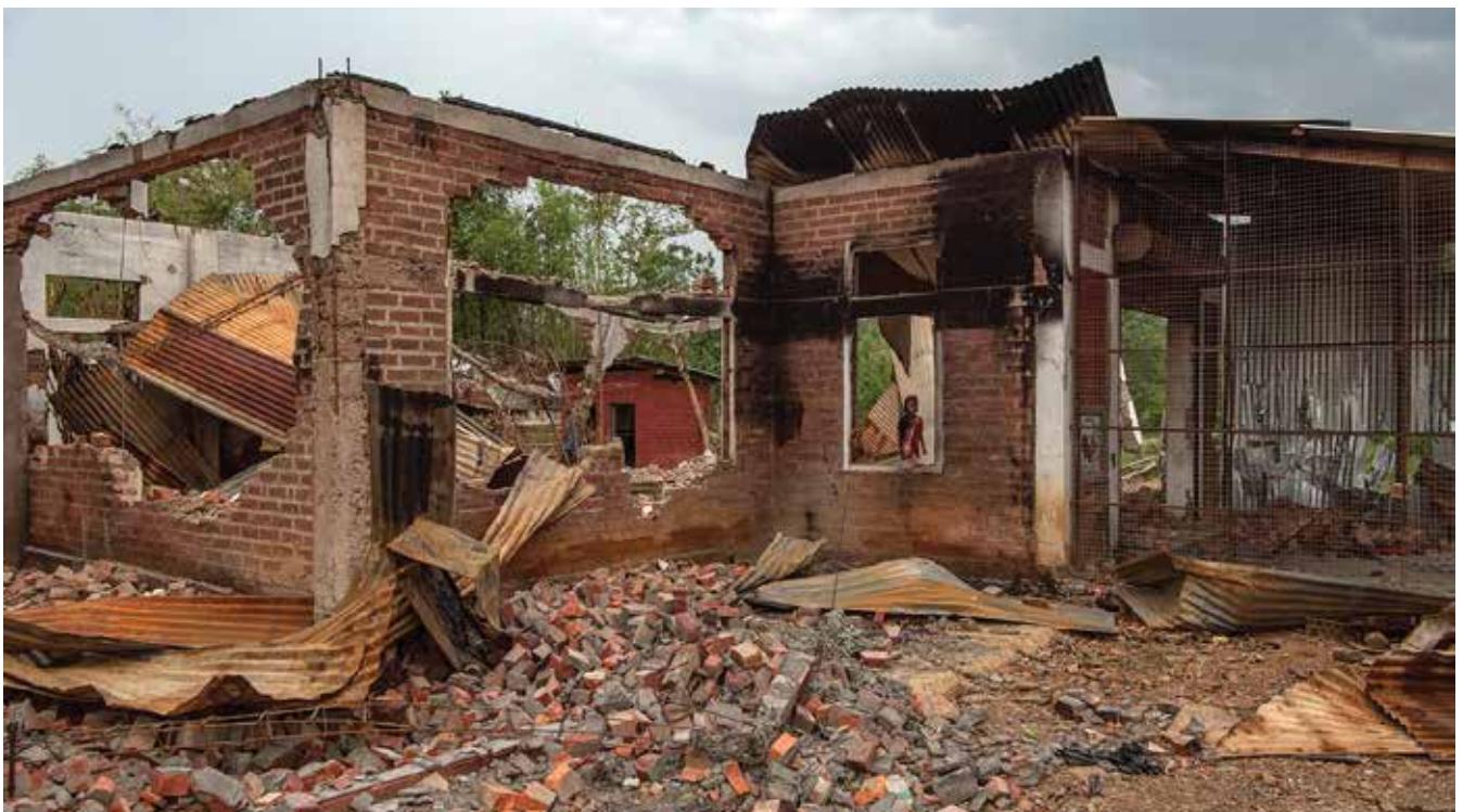
Burnt down houses in churachandpur district, on 31 May
